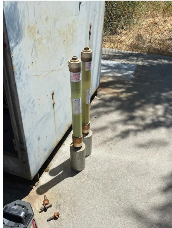
Fuse replacement at Merritt
