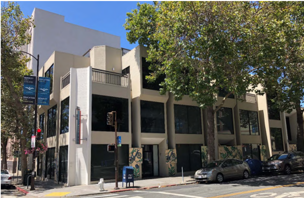
Figure 4 2118 Milvia Street, South and East Elevations, Facing Northwest
