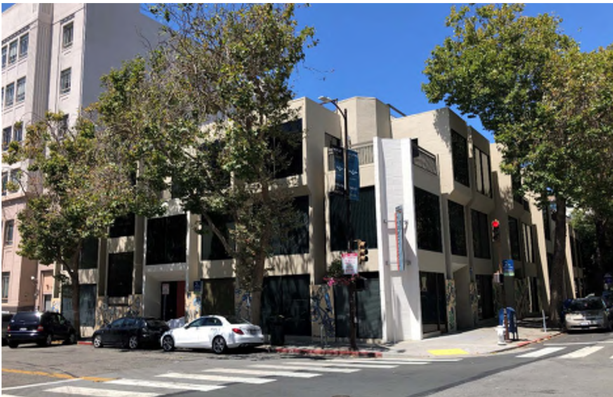
Photo 2. View of project site looking northwest from the Milvia Street and Center Street intersection.
