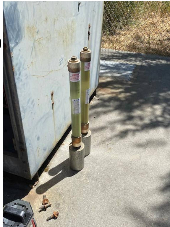
Fuse replacement at Merritt
